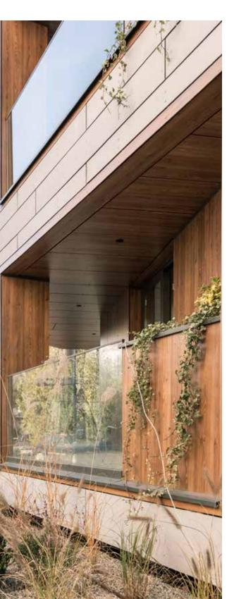
The layers of kraft and decorative paper are impregnated with thermosetting resins, dried and pressed under high pressure at high temperatures to obtain a panel with exceptional properties, in compliance with the European standard EN 438.
